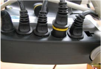
Connected the motor to the control unit.
